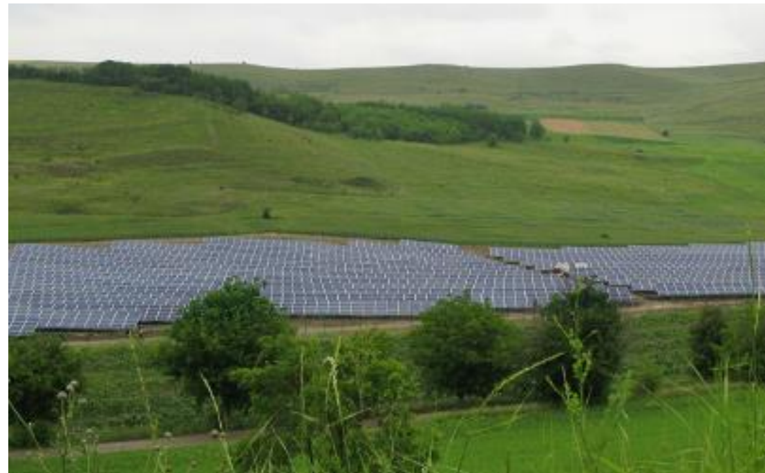
The German PV company built the facilities for a Romanian private investor on almost 19 hectares în the county of Mures
